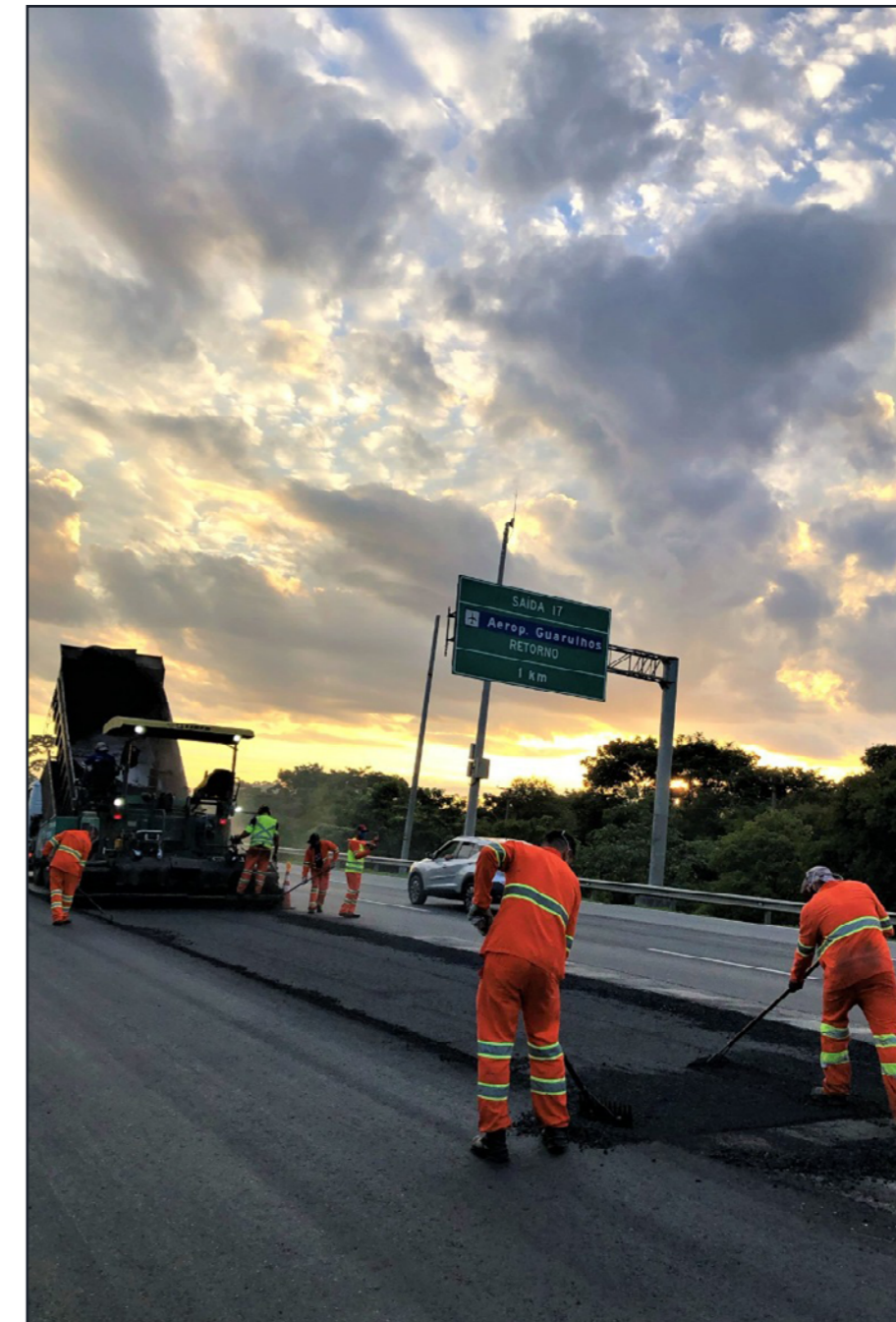
Works at SP-070 Consortium
